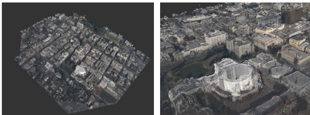
(a) Berkeley overall view
