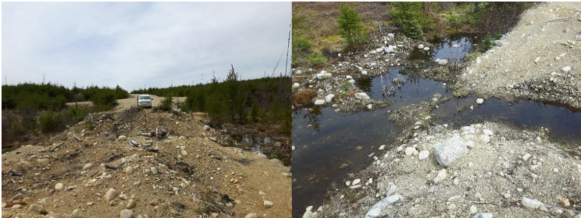
Figure 5. Left, the extent of excavation of the water crossing and road berm preventing road vehicle access. Right, evidence of access beyond the water crossing removal and berm. Both photos were taken as part of the study area assessment, May 15th, 2017.
