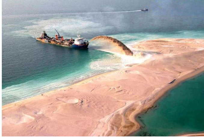
Figure 1.1 Palm Islands construction in Dubai
