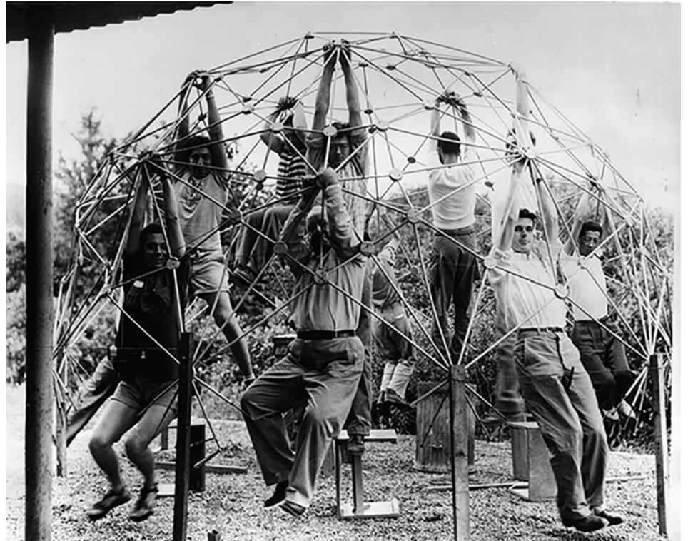
[Fig. 6]. Students constructing the geodesic Dome, Black Mountain College, 1949.
