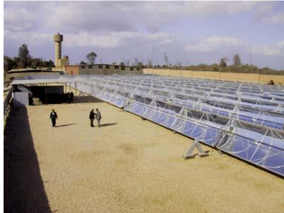
Figura 15 - El NASR Pharmaceutical Chemicals, Egypt. Installed capacity: 1.33 MWth. (From Fichtner Solar GmbH, 2005 Germany. With permission.) ( http://www.aee.at/aee/images/Bilder-fuer-Zeitungen/2005-03/images/01_4.jpg )
