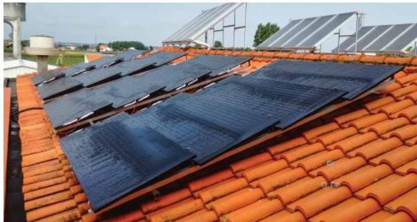
Figura 17 – Sistema solar termodinâmico instalado numa IPSS ( http://www.energie.pt/en/all-news/item/420-sanitary-hot-water-ipss )
