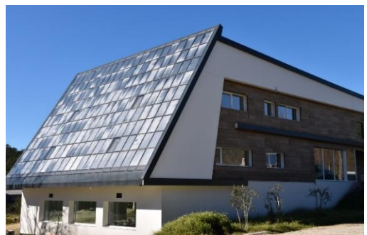
Figure 2 - Actual size façade with 200 square meters in operation at the Portuguese Sustainability Centre (CPS), Campia, Portugal (Coordinates: 40.652482, -8.209533).
