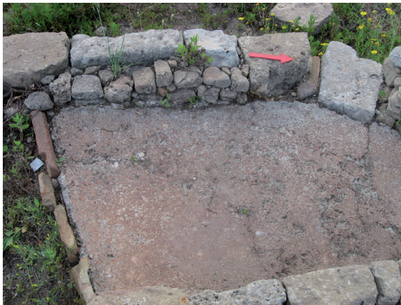
Fig. 2 – Megara Hyblaea. Cement floors: broken terracotta concretes (four top pictures); limestone mortars (four bottom pictures)
