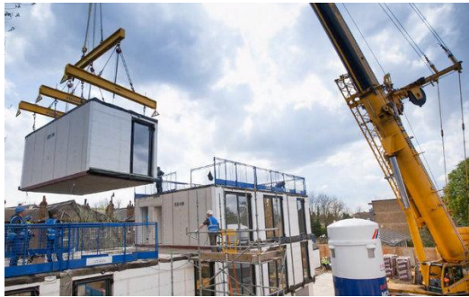
Fig 1: Installation of Modular Housing Source: Lawrence (2017).
