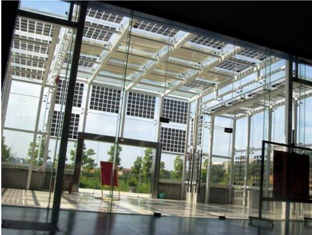
Figure 1.1 Building Integrated Photovoltaic
