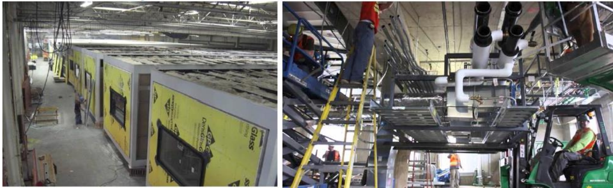
Figure 1. Prefabricated building modules and MEP pipe racks (Smith, et al., 2015)
