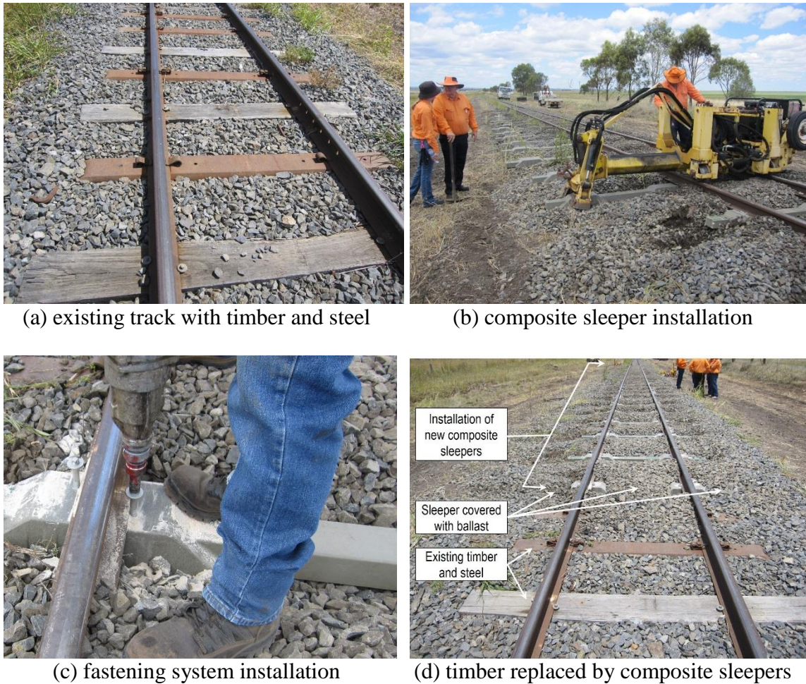
Fig. 5: Installation of composite sleepers replacing existing timber
