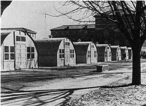
WHEN IT RAINED, THEY CLANGED. Metal Quonset huts served as auxiliary classrooms for the late forties’ deluge of students. But when it rained, the din on the metal made hearing lectures difficult.
