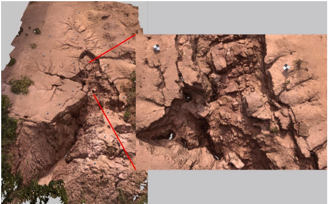
Fig. 5. Dense point cloud showing the 3D reconstruction of complex topographic areas inside the gully.
