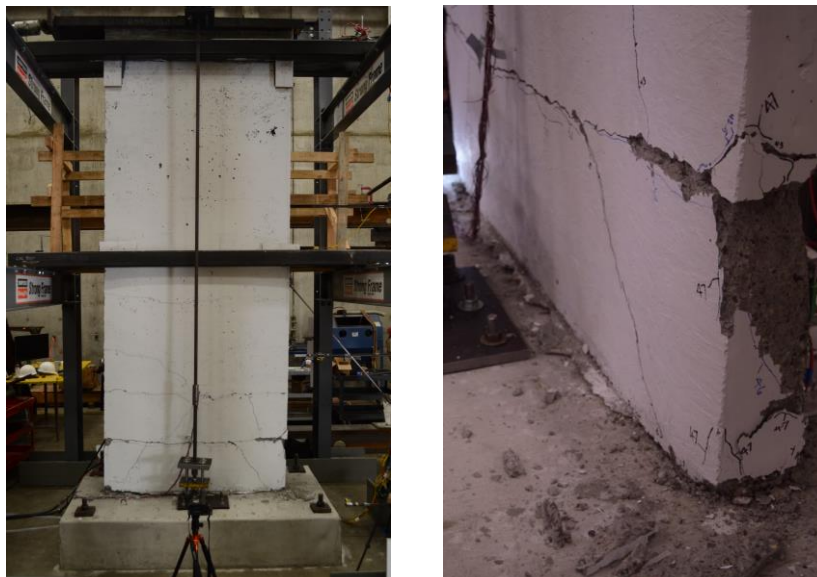
Figure 6. Final damage state of wall: (left) overall, (right) north wall end zone
