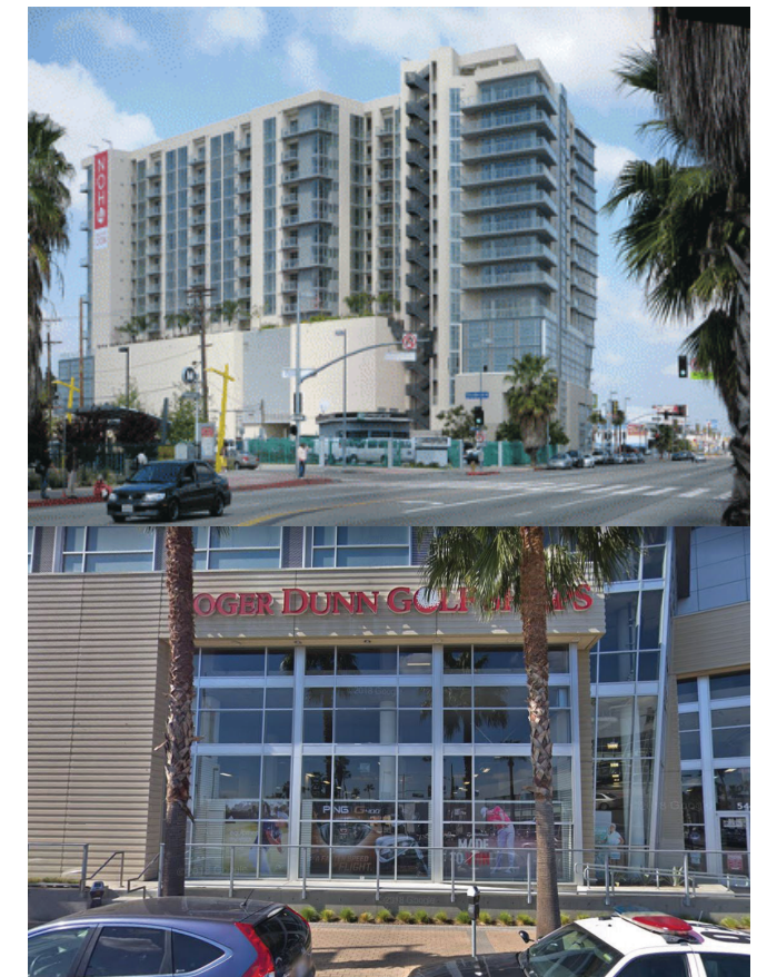
Figure 4.2.4. NoHo 14 Apartments and Roger Dunn Golf Shops [2]
