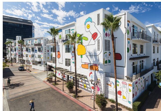
Figure 4.2.7. Lofts at NoHo Commons Apartments [5]
