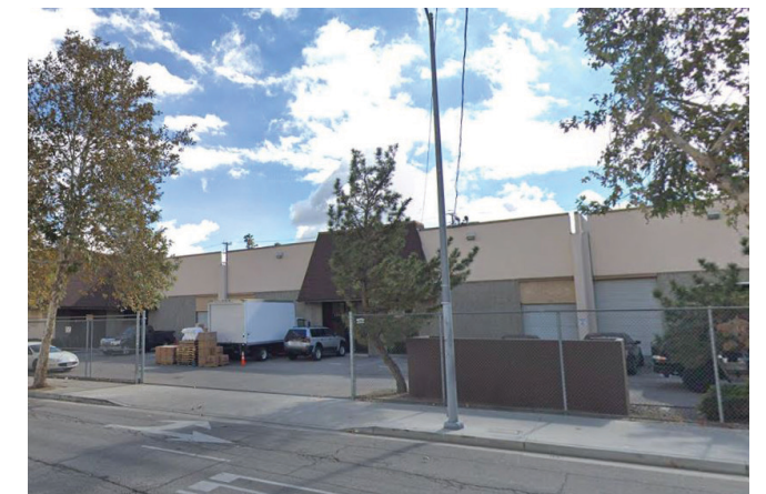
Figure 4.2.5. Warehouse on Chandler Boulevard (westbound) [3]
