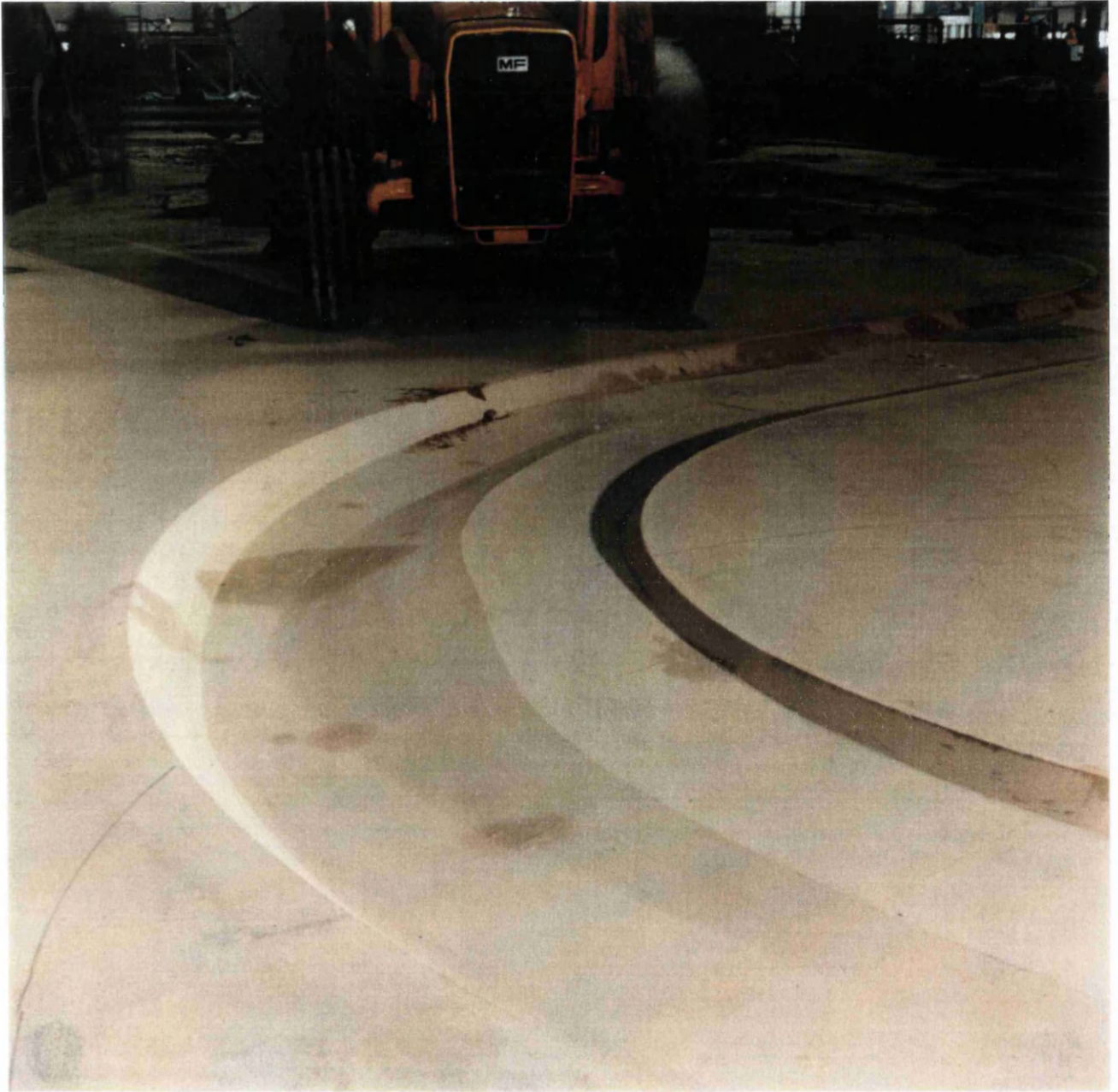
Fig (3.21) - A View of the Bend Region of the Natural Meandering Channel( sinuosity 1.37), after Construction. S.E.R.C. Series B.
