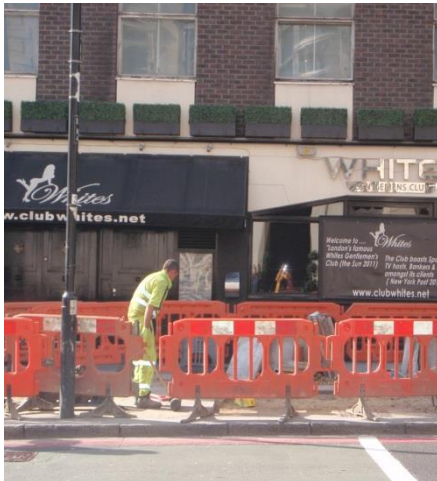
Figure Twenty Seven: Construction work, London Wall
