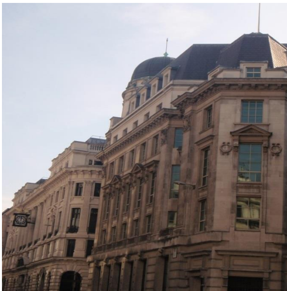
Figure Fourteen: Victorian buildings on Gracechurch Street
