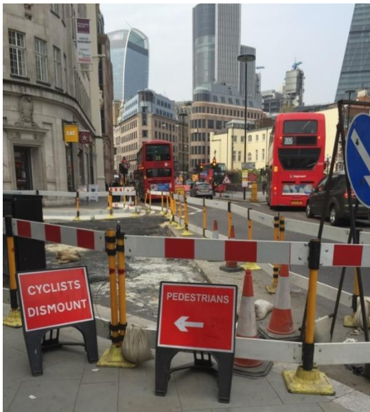
Figure Thirty One: Construction work near Aldgate, Sunday afternoon
