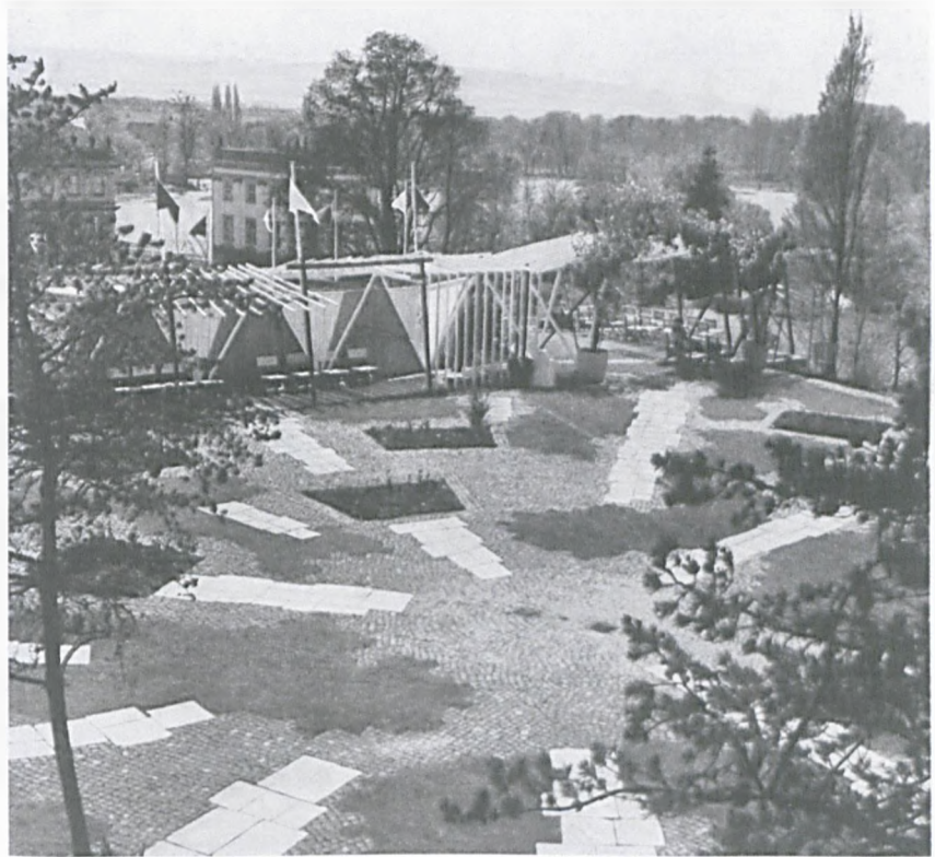
Fig. 92) Entrance square with experimental lightweight architecture at the Federal Garden Show 1955 at Kassel by Hermann Mattern, stone slabs, pavement and macadam. Baukunst und Werkform , 7 (1955), 439.
