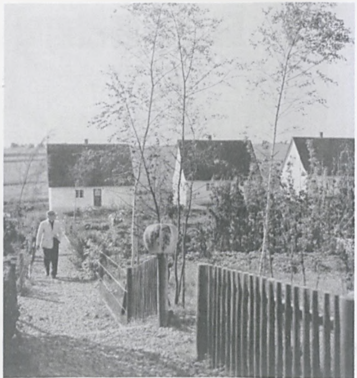
Fig. 135), 136) Settlement 'Auf der Brücke' at Rottweil, by Mattern and Paul Schaeffer-Heyrothsberge, architect, 1936. In publications about it the potential of communal spaces for child's play was emphasiscd. Plan courtesy: Architekturmuseum TU Berlin, F 2647. Photo: Hermann Mattern (ed.), Die Wohnlandschaft (Stuttgart: Hatje, 1950), p. 71 (the photo may show a similar project completed with Schaeffer-Heyrothsberge at Dallgow).
