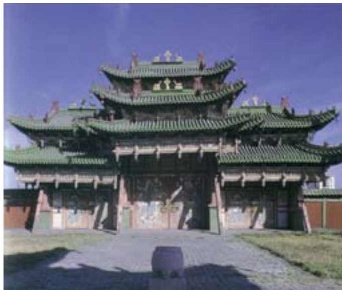
FIG. 27. Ulaanbaatar. Andingmen (detail): front of the main gate in the ceremonial gate complex, completed in 1919. (Source: Tsultem, 1988, Pl. 71.)
