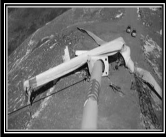
Figure 75 Total turbine collapse in Gansu at the North Bridge wind farm. (Source: Lin, Y., 483)
