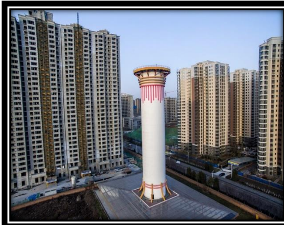
Figure 88 Functioning SALSCS prototype tower in X'ian
