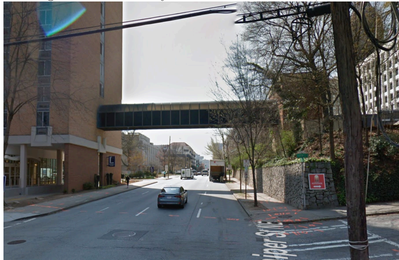
Figure 28: Walkway over road at Route 1, Turn 3.
