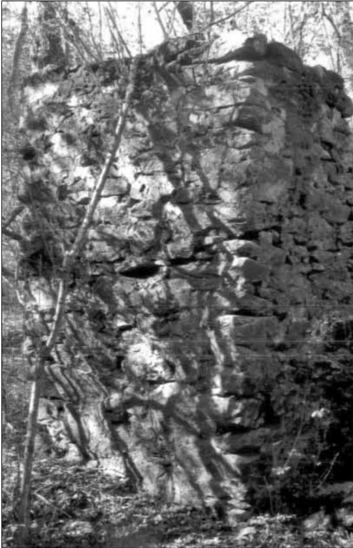
Figure 10. Unidentified Structure, Troup Factory, LaGrange, Georgia.
