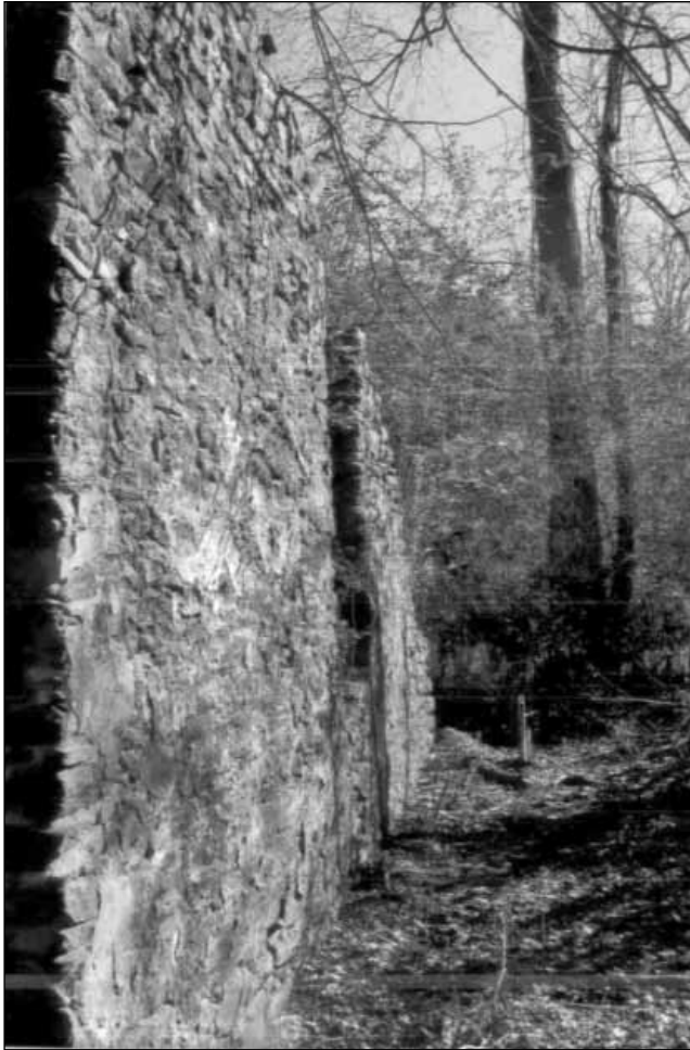
Figure 7. Walls of the Picker Room, Troup Factory, LaGrange, Georgia.
