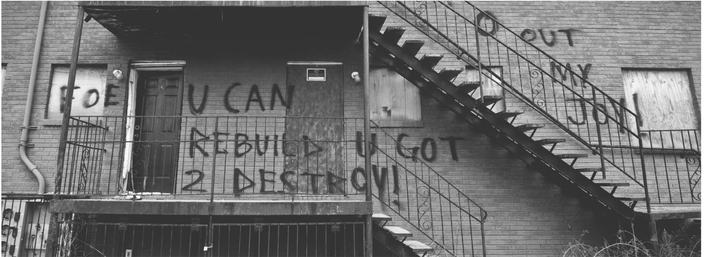
FIGURE 2.10 - BEFORE YOU CAN REBUILD YOU HAVE TO DESTROY
