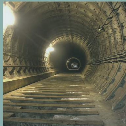
FIGURE 48 - ROUGH SUBWAY TUNNEL
