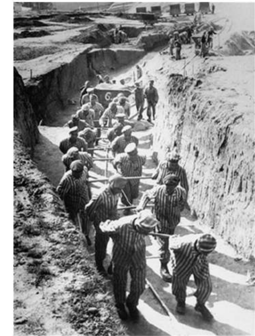
FIGURE 1.7 - SLAVE LABOUR AT STONE QUARRY
