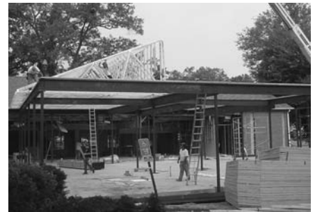
The steel frame construction begins.
