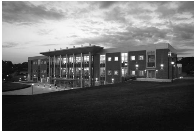
The Library Technology Center of North Georgia College and State University in Dahlonega (Photo courtesy of The Whiting-Turner Contracting Company)
