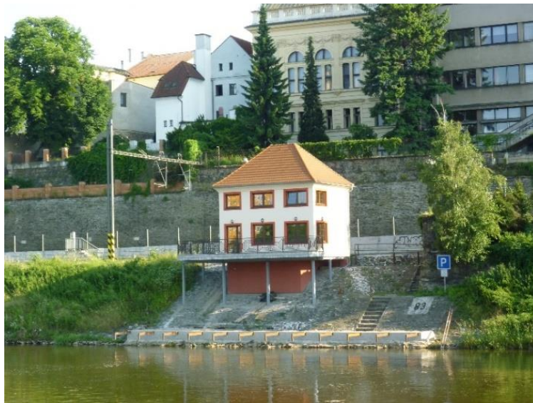
A previous water pumping station in Kolin, which is now being converted into a river side restaurant/bar complete with a boat dock, Summer of 2014, Photo by author.
