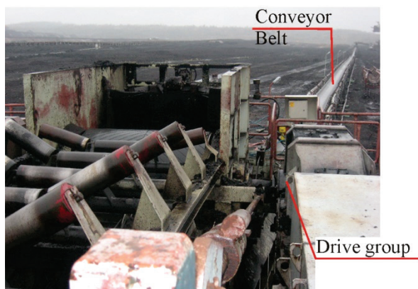
Figure 1 Conveyor belt TS305-drive group
