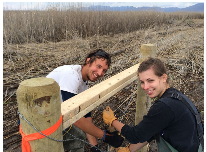
Fence installation for containing cattle in target areas. Image: Karin Kettenring
