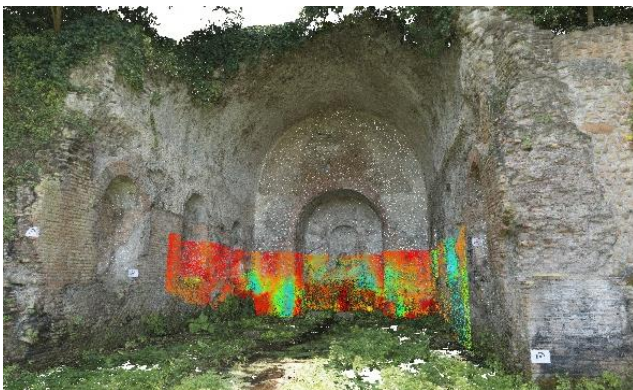
Figure 7. RGB point cloud integrated with IRT data
