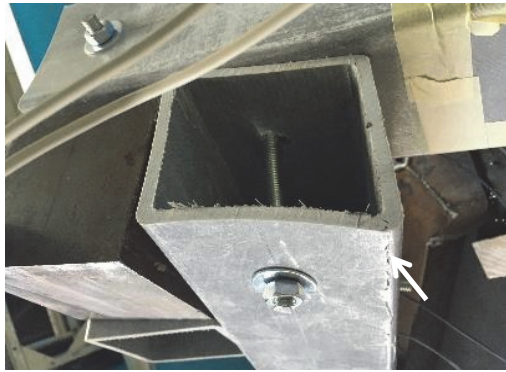
(a) Web-flange junction fracture/tearing
