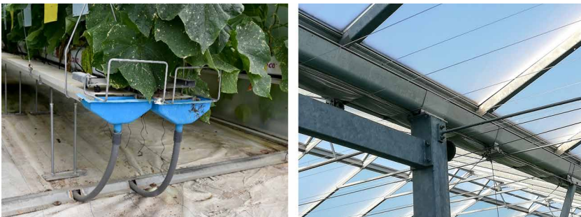
Figure 2 Collection of water drained from the cultivation system after irrigation (left) and water transpired by plants as vapour and successively condensed on greenhouse roof (right).
