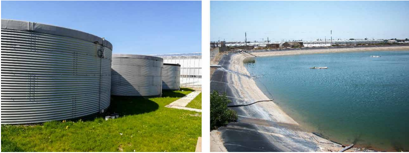
Figure 1 Examples of water silos (left) and lined water storage (right) for the collection of rain and/or drainage water.
