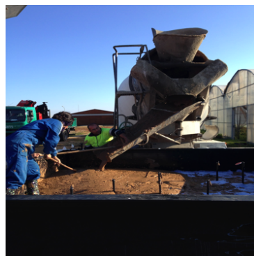
Figure 5.43. Pouring the slurry in the container.
