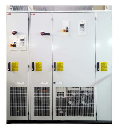
Figure 2.7: ABB ACS 800 controlling panels.
