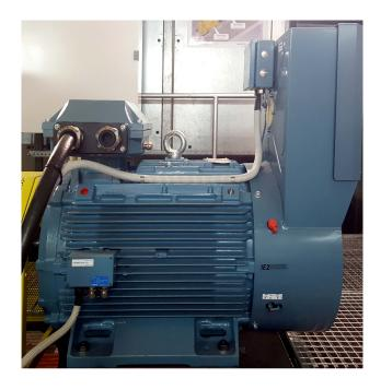
Figure 2.5: ABB Electric Motor 90 kW.
