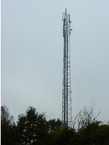
Picture 1.2. – Mast for mobile communication with several antennas in it. Photograph by author.
