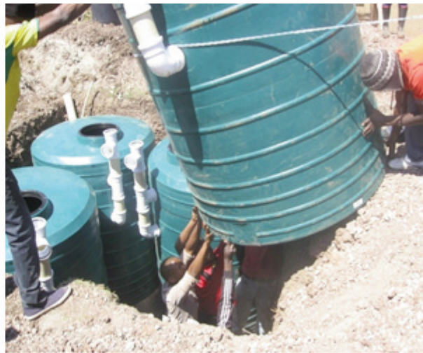
Placing digester tanks in side hole
