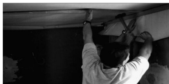
Figure 10: Installation in progress at the CSIR
