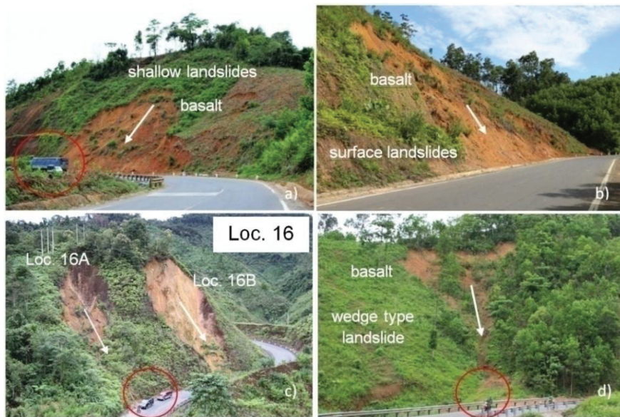
Fig.4. 22 Surface landslides, shallow landslides (photos a, b) and the wedge type (photos c, d) on HCMR, around KhamDuc town
