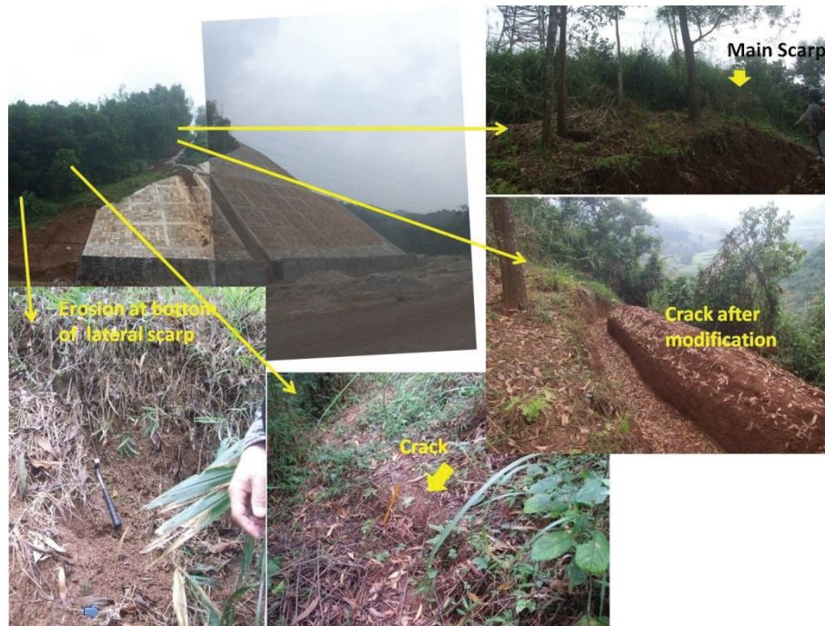
Fig.4. 80 Some micro features of Km90landslide (photos taken in Aug. 2013)
