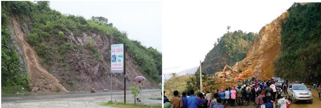
Fig. 3. 8 Complex landslides on HCMR (shallow landslide with earth flow) and NH6 (slump-earth flow with rock fall debris)
