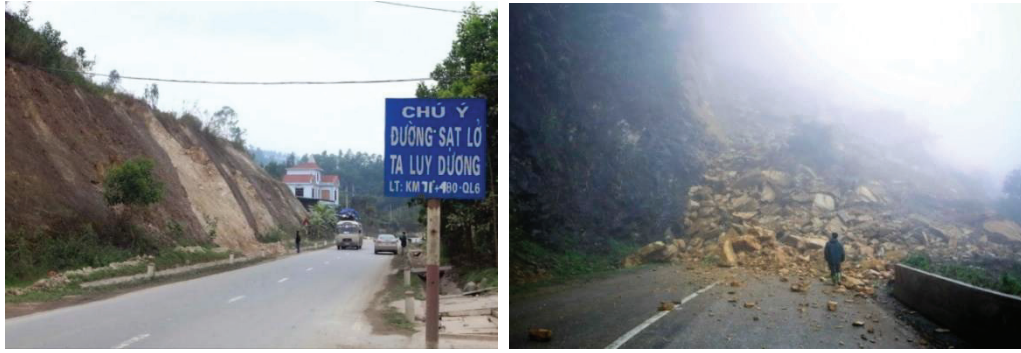
Fig.2. 4 Landslide warning board at Km71+480 and a landslide at Km138+750 along NH6
