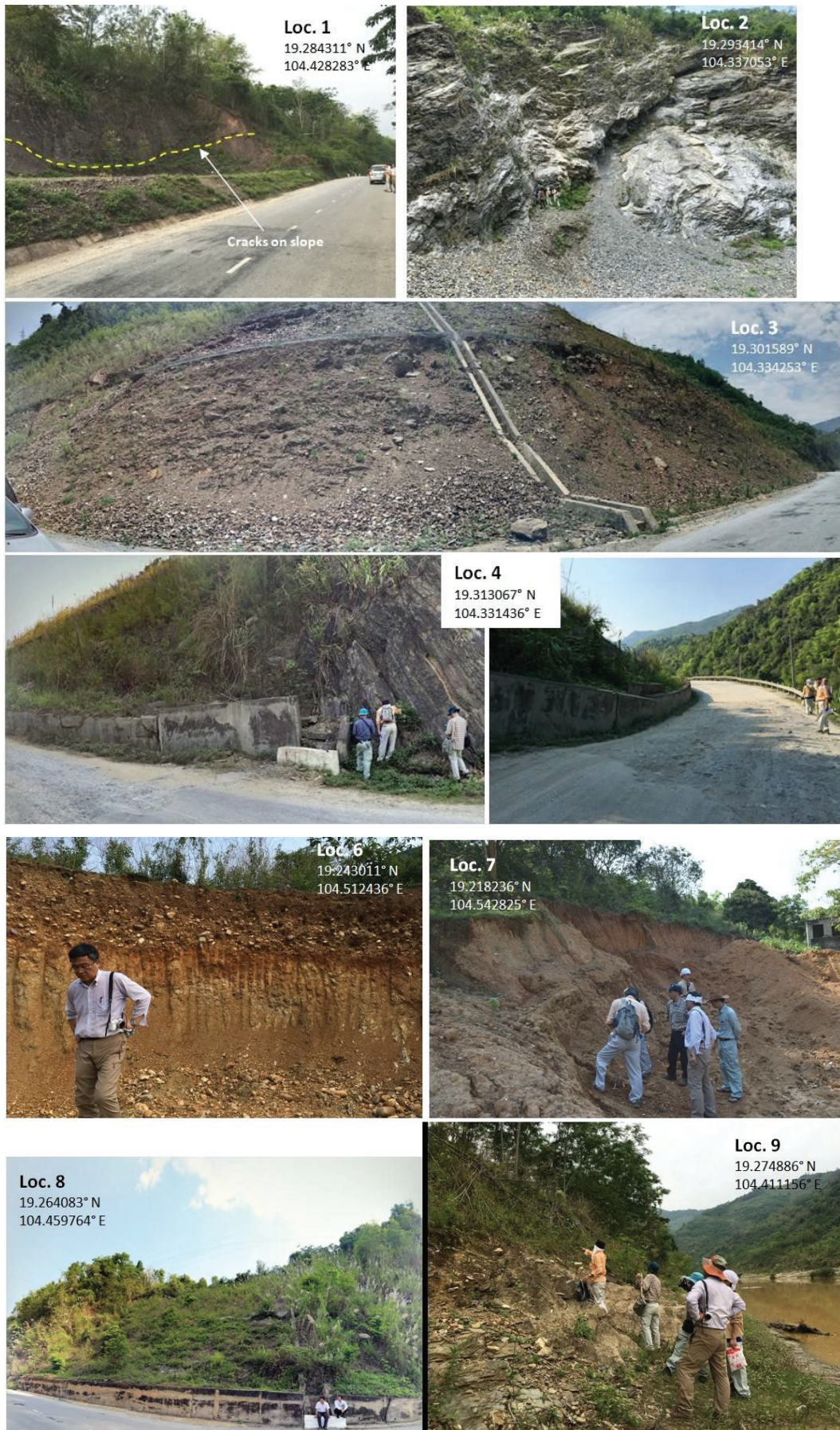
Fig.4. 27 The overview photos of landslides along NH7
