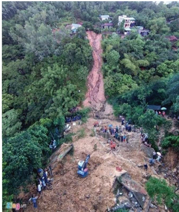
Fig. 1. 8 A landslide in Ha Long city, 9 people buried under hundreds of tons of rock ( zing.vn )
