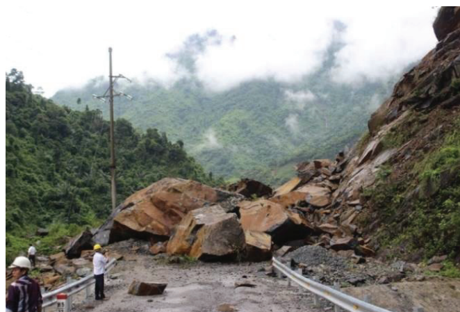
Fig.2. 8 Landslide caused serious traffic congestion on National Route 279
