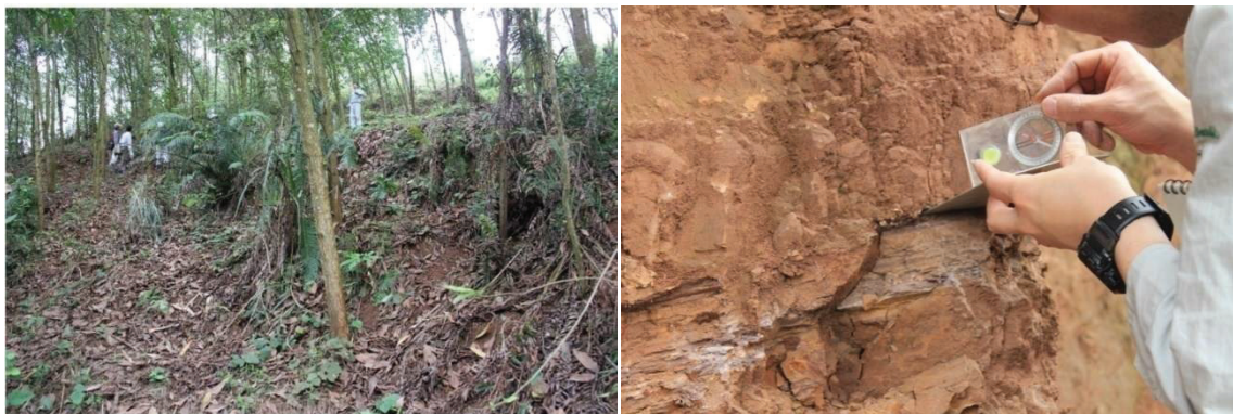
Fig.4. 81 Some distinctive shallow landslide characteristics around Km95 landslide (left) and Relatively fresh rocks at nearby the landslide area (right)
