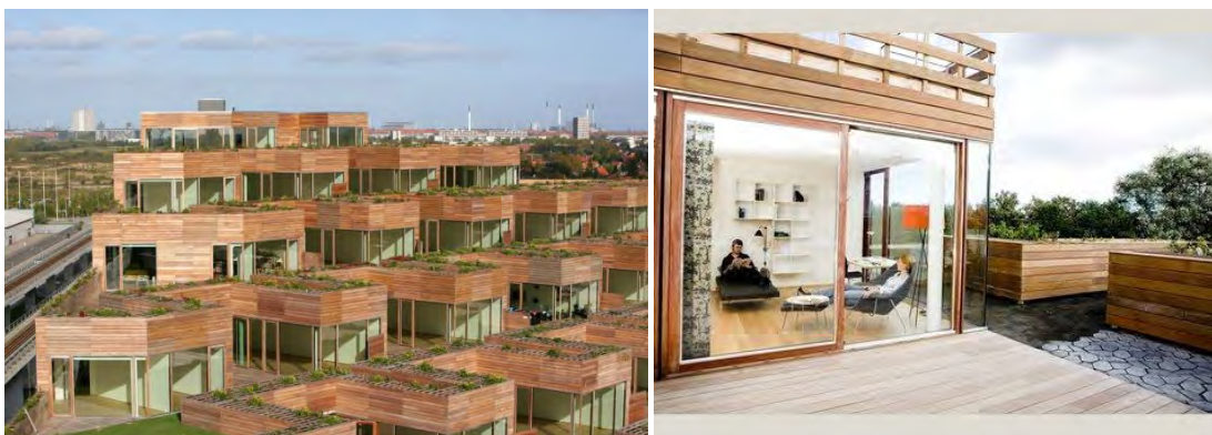
Figura 42 e 43 – Autor: Ulrik Jantzen - "Fotografias mostrando os jardins existentes na cobertura." (Fonte: http://www.archdaily.com/15022/mountain-dwellings-big/553962616_big-02/ ); (Fonte: http://www.worldarchitecturefestival.com/clientUpload/images/project/large/MTN%20PHOTO%20ULRIK%20JANTZEN%20%284%29%2Ejpg )
