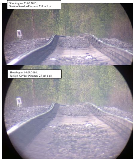
Pic. 6. Relative depressions of the track at the 25 th km of the Kovdor–Pinozero section.
