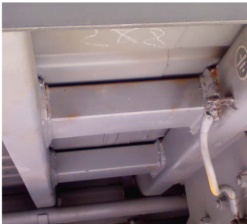
Pic. 4. Car frame reinforced with longitudinal beams.
