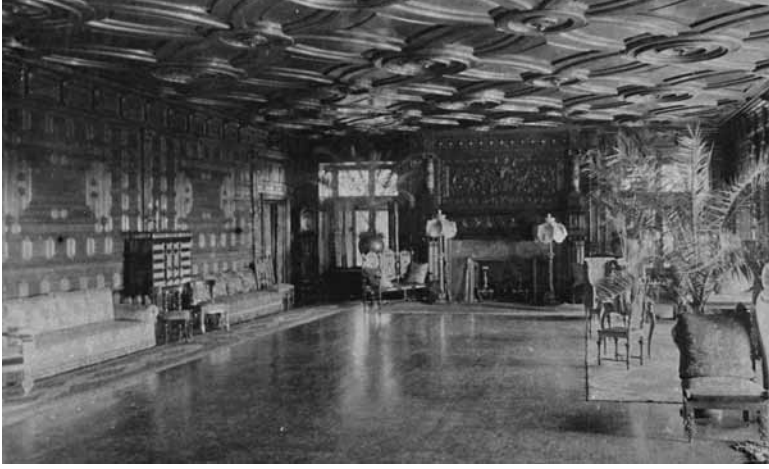
The ballroom. Its massive oak ceiling was suspended on chains hung from beams in the attic above the third-floor. The windows on the right looked out on Lake Mahkeenac.
