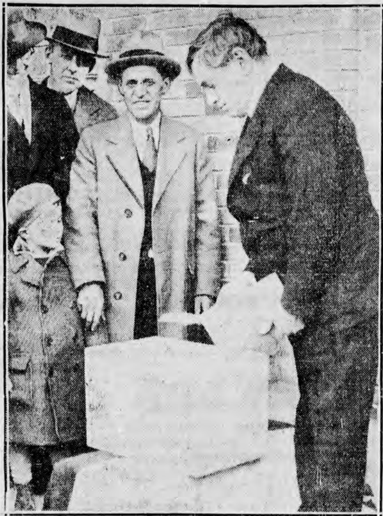
LAYING L STREET BATH CORNERSTONE
