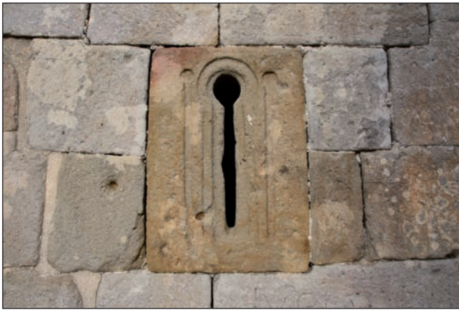
Fig. 6. Apse window of San Julian and Santa Basilisa church (Aistra, Zaldondo, Alava)
