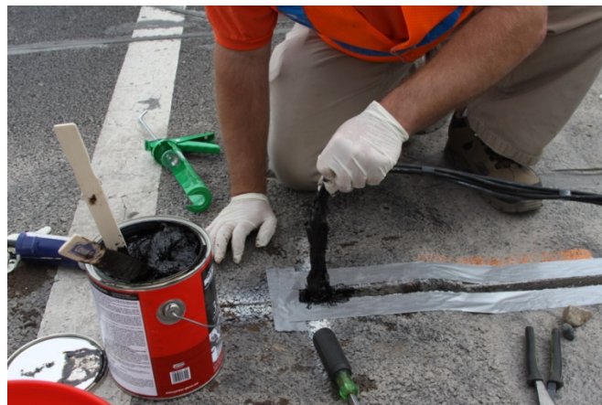
Figure 3. Installation of temperature probes.
