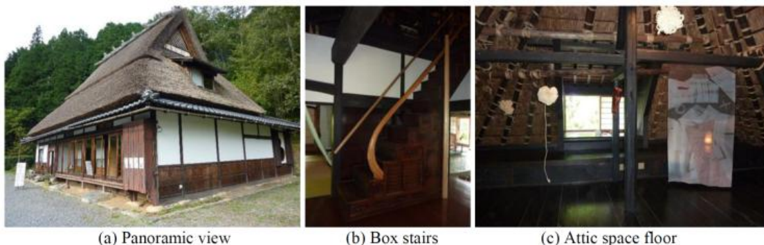
Photo 1. One-storey thatched roof wooden structure
