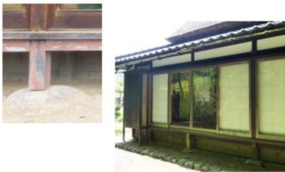
Photo 2. Post erected on a foundation stone
