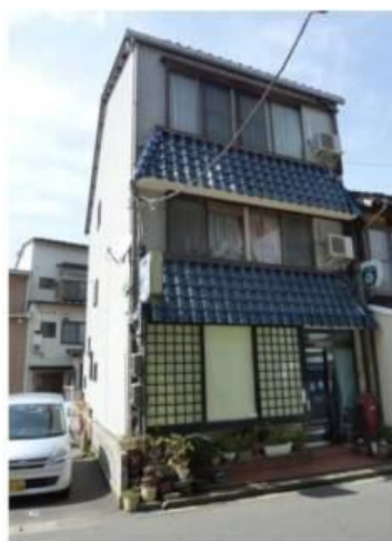
Photo 1 Elevation view of 3-story wooden house
