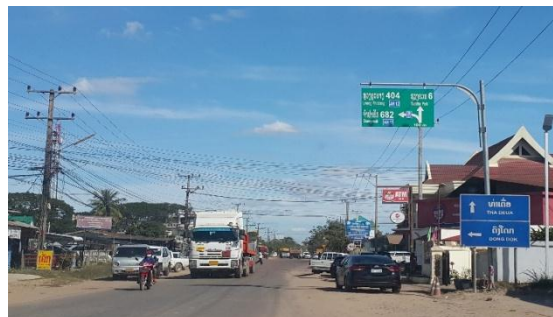
Figure 6. Road Infrastructure in Thanaleng
