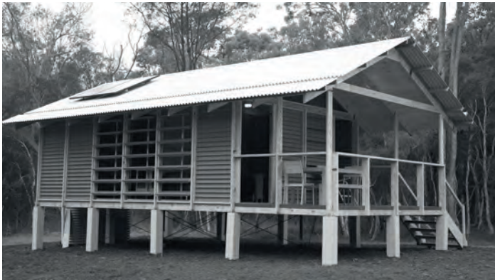
Devastation caused by Cyclone Pam in Vanuatu, March 15, 2015 (top) and a NevHouse prefabricated home made from recycled plastic, offering solutions (bottom) (Courtesy of Jessica Williams)
