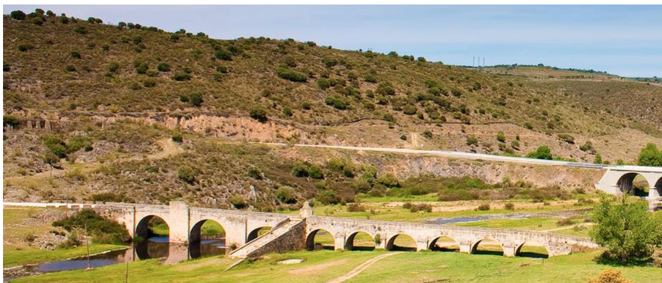
Figure 1. Photograph of the Bridge.
