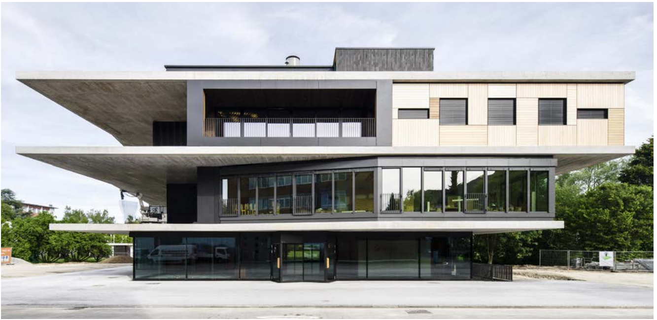
Figure 2. Outside view of the NEST building with the Backbone and two units: Meet2Create on the first floor and Vision Wood on the second floor.
